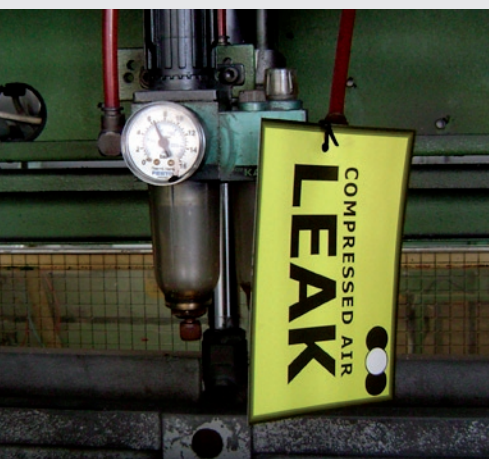
Leaks can account for the biggest losses in compressed air systems
