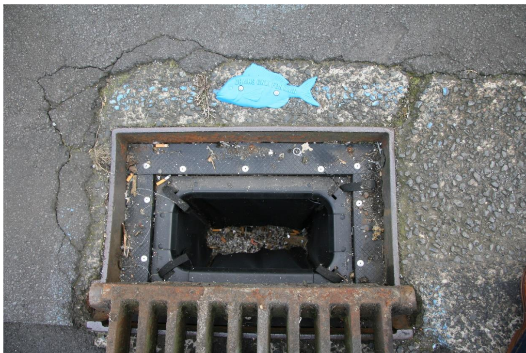
Figure 5. A LittaTrap in place on a manufacturers site, with collected material caught by the filter
