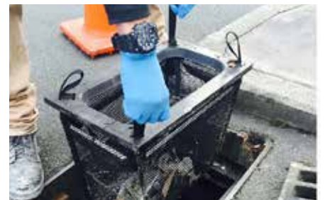
Stormwater catchpit filters such as this one are an easy, cost-effective solution
